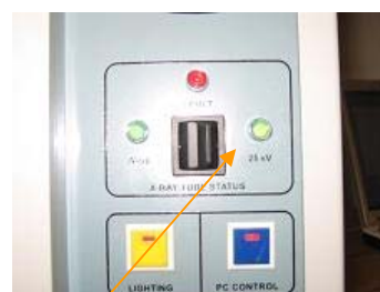
Warning: Must not operate the equipment until 25kV green LED light is stable
